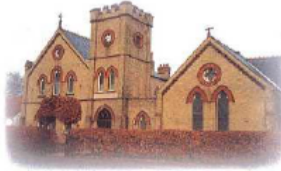
A Grade II listed historic building
